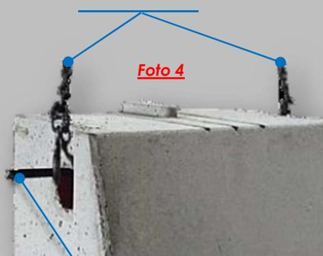
Barra in ferro  $\geq \varnothing 18$
